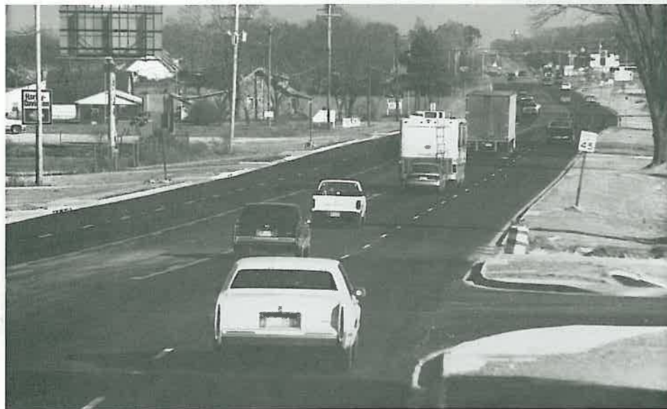
Newly widened section of Highway 412 at Tontitown
